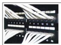
The photo above shows a typical category-5E patch panel with patch cables connecting each network segment to a port on the Hub.
